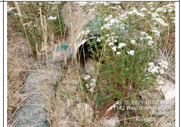
Inlet to Outfall #10
