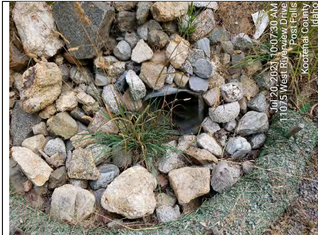
Inlet to Outfall #11
