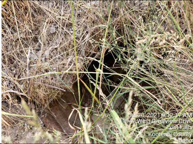
Inlet to Outfall #7
