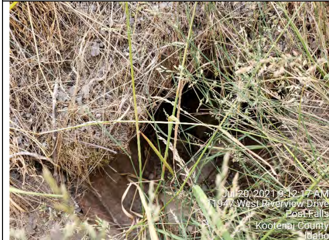
Inlet to Outfall #7
