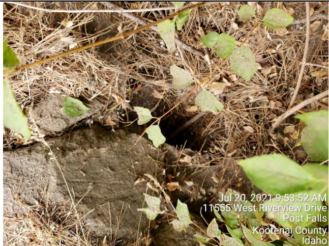
Inlet to Outfall #9
