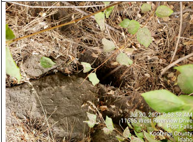
Inlet to Outfall #9
