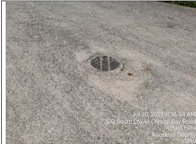
Inlet to Outfall #5
