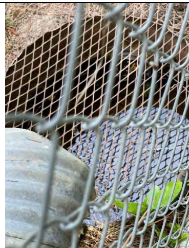
Inlet to Outfall #8
