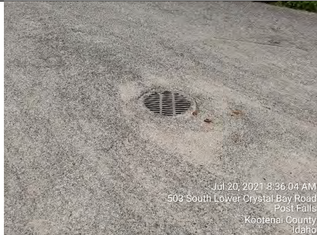
Inlet to Outfall #5
