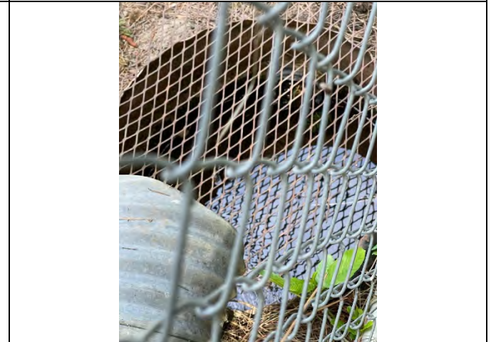
Inlet to Outfall #8
