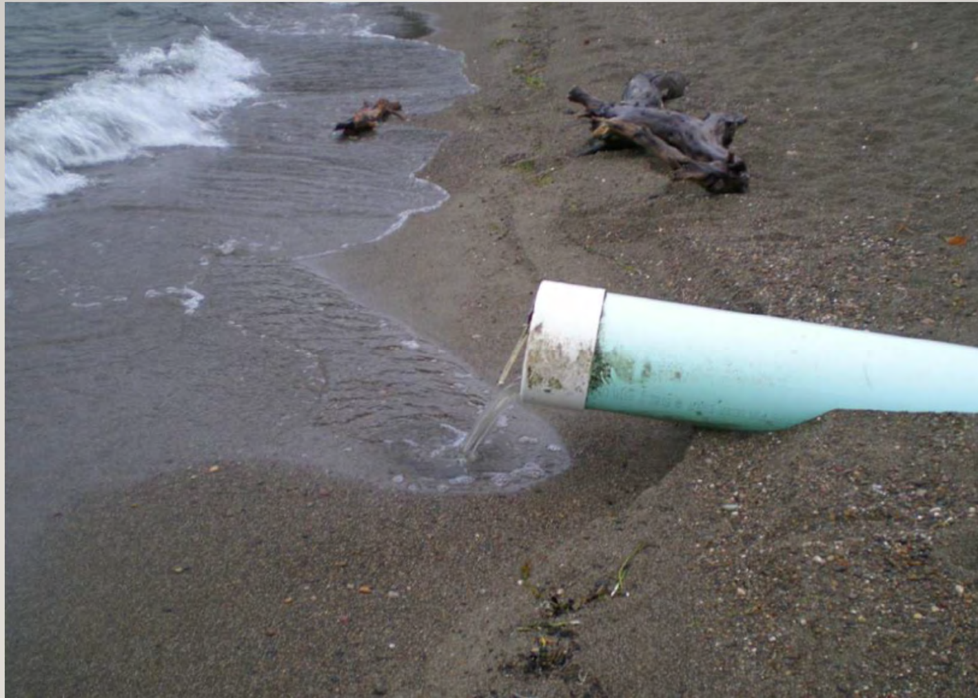
Sanders Beach Outfall
