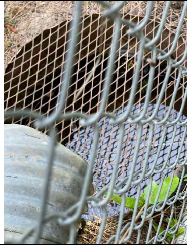
Inlet to Outfall #8
