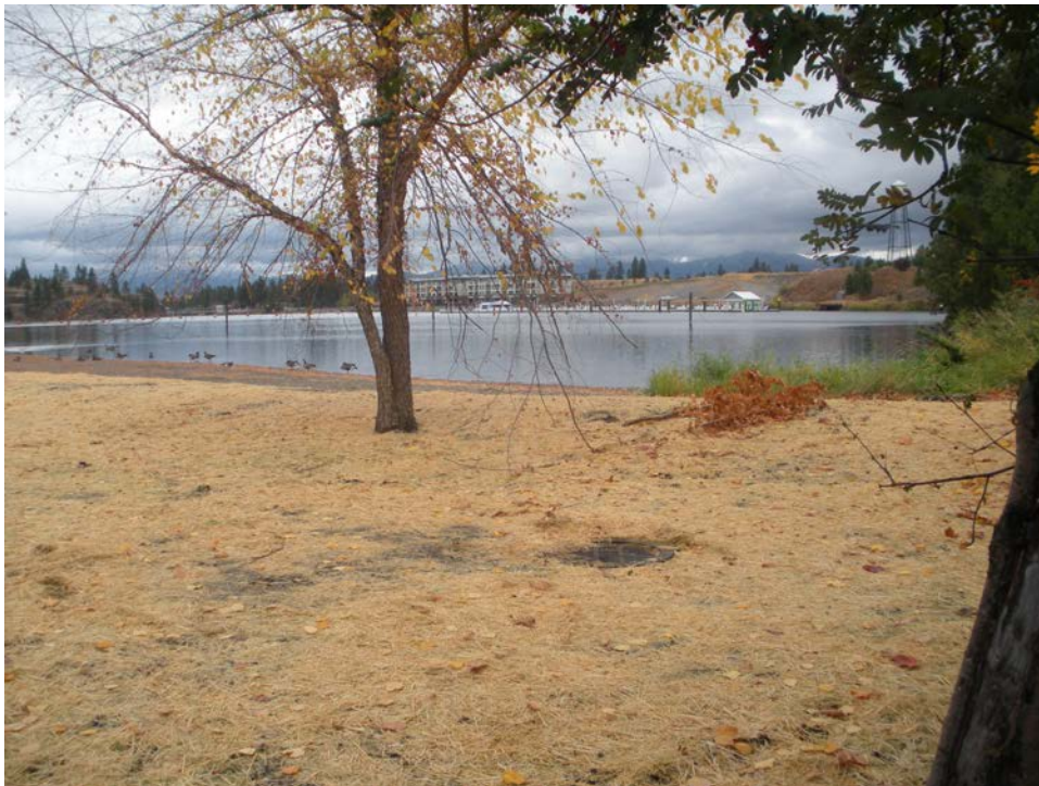
Photo 2: Spokane Street Drainage Improvements (10/23/12) New Swale with Dispersed Straw West of Catch Basins/Outfall #6
