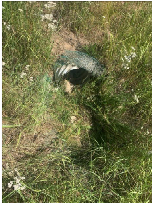
Figure 4: Outfall 10 Culvert (2022 Dry Weather Inspection)
