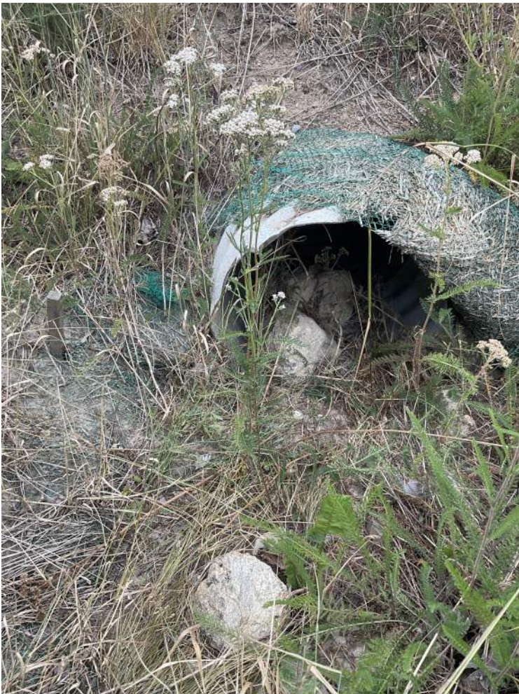
Upstream Culvert Assessed:
