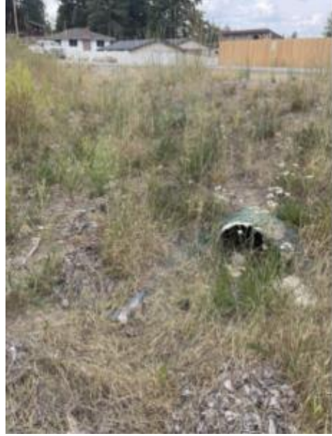
Outfall 10 (inlet, outfall submerged)
