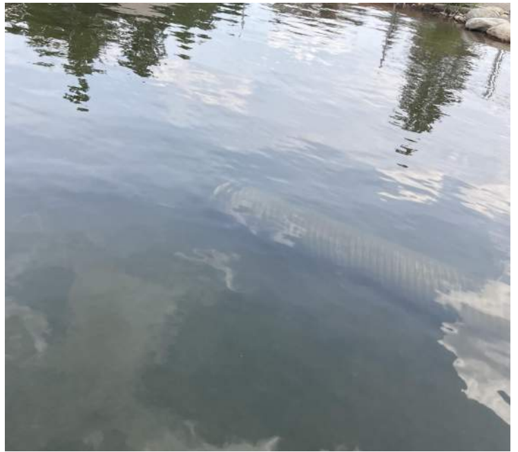
Outfall Fully Submerged in Spokane River:
