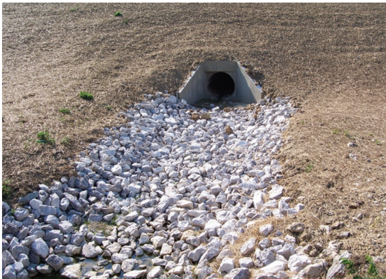
Figure 17. Make sure inlets, outlets, and slopes are well stabilized before leaving the site and filing your "Notice of Termination" for ending permit coverage.
